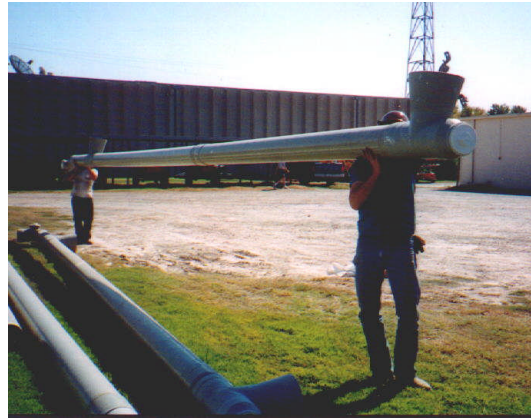
Figure 1 – Two men carry 40' of 8" pipe in Topeka, Kansas
